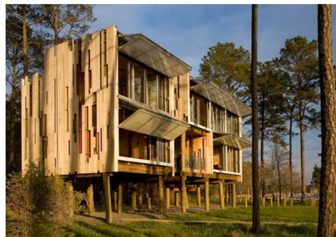
Fig. 6. Loblolly House, S. Kieran 2007, Taylors Island, Maryland, USA
