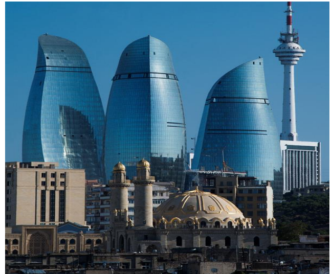
Fig. 2. Flame Towers, Baku, Azerbaijan, HOK International, 2012
