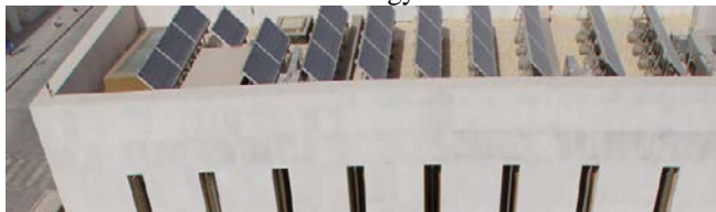
Fig. 13. Shows the solar panels on the mosque's roof [27].
