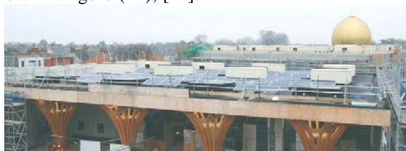
Fig.11. Shows the solar panels and solar heaters on the roof of Cambridge mosque [25].
