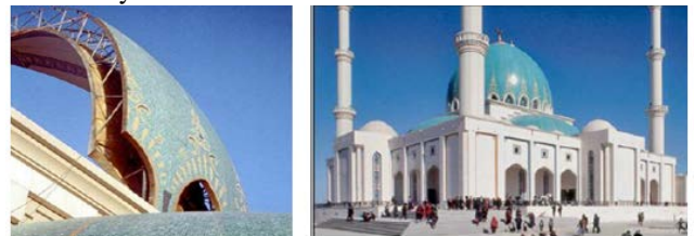
Fig. 30. Shows double layers dome in Goktepe mosque [43].
