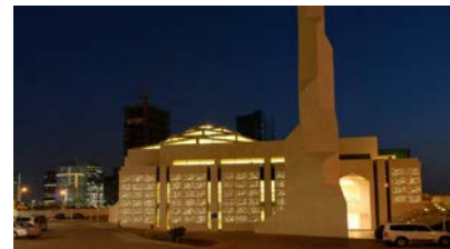
Fig.37. Shows transmitting concrete in façade of Al Aziz mosque in Abu Dhabi [55].
