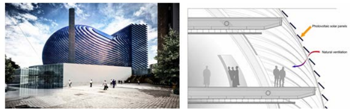
Fig. 29. Shows Solar panel dome in Kosovo mosque [42].
