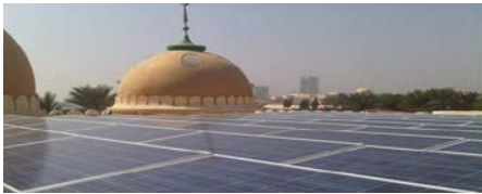
Fig. 20. Shows the use of photovoltaic solar panels on the roof of Ambar mosque in India, [35].
