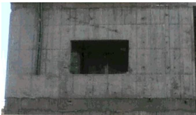
Figure 1: Concrete shear wall with opening (Iran; Semnan 2011)
