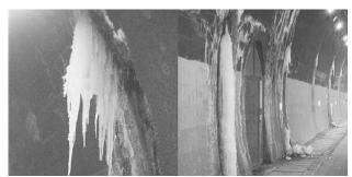
Figure 2 The lining freeze of a tunnel
