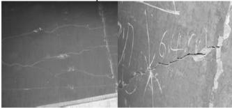
Figure 1 lining crack of a tunnel (Mined out area in the low of the tunnel)
