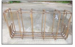
Fig. 1. Reinforcement cage for deep beam
