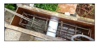
Fig. 3. Concreting for deep beam
